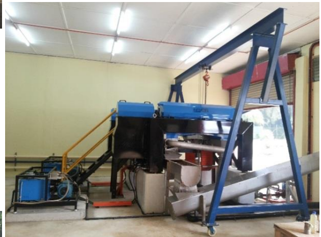
Package 2: Construction And Completion of Sg. Sayong Sludge Treatment Facility And Associated Works
