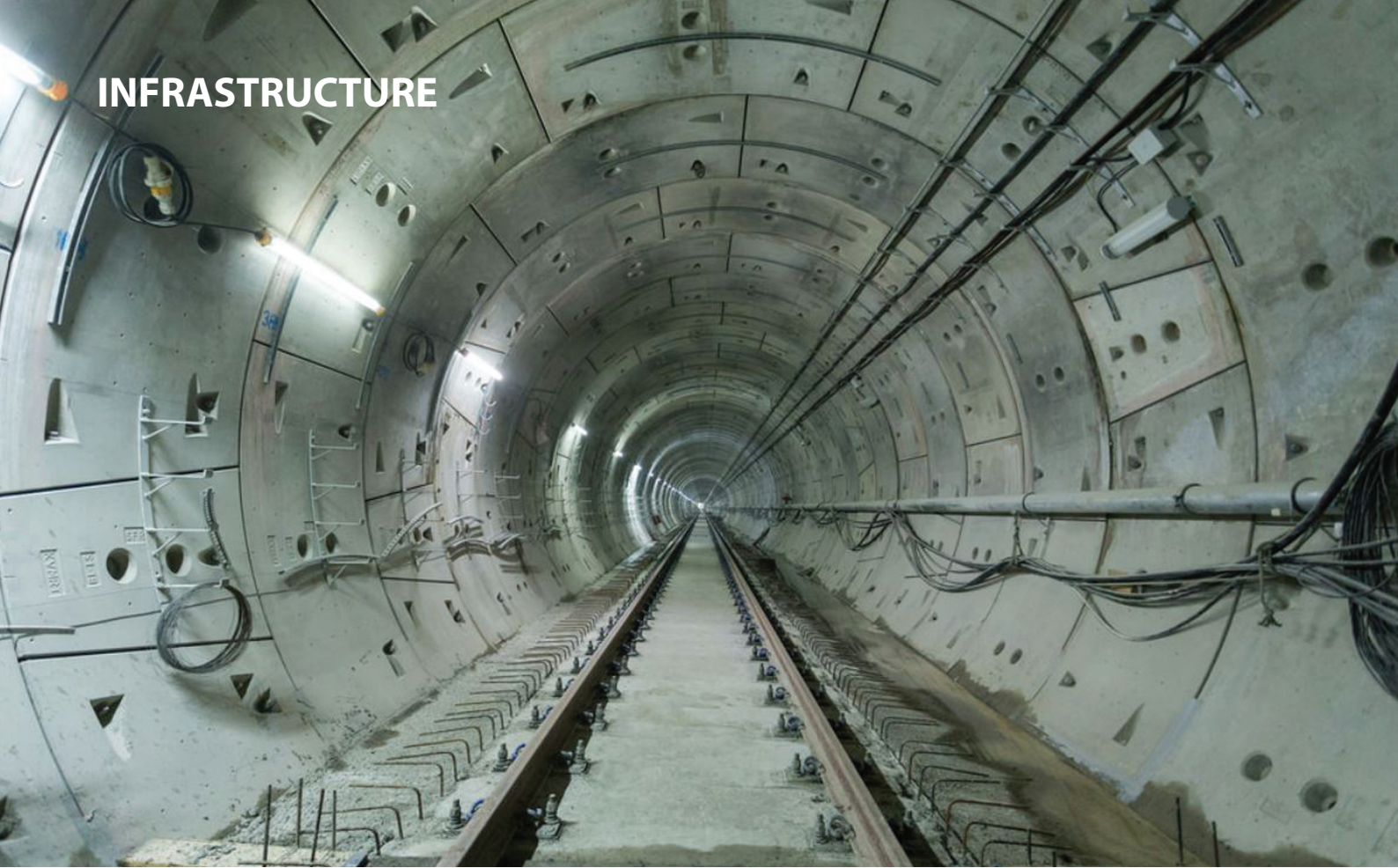
Completed tunnel lining for MRT Line 1.
