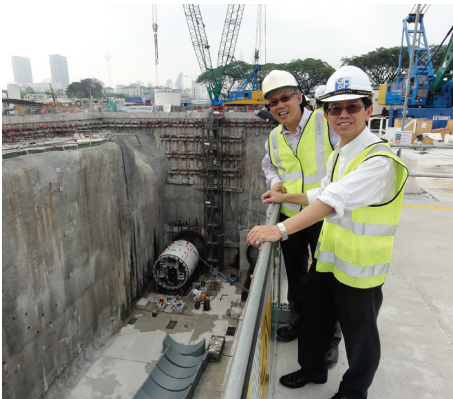
Site visit by Dato' Ir Dr Gue S S (CEO) (right) and Ir Dr Tan Y C (Project Director) during preparations for TBM launching.
