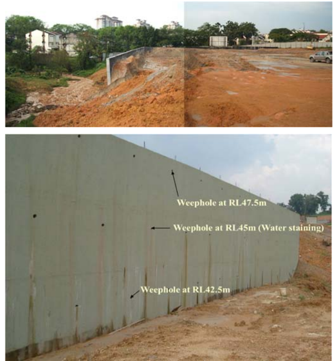
Figure 1 Overall Site Condition and Evidence of Rising Groundwater Level in the Wall Backfill
