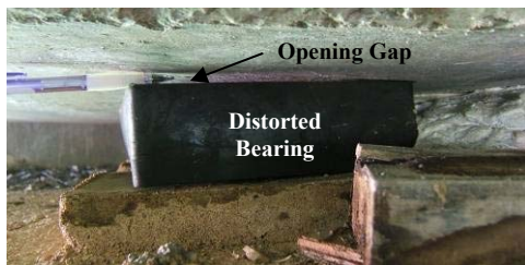
Figure 15 Shearing distortion of rubber bearing
