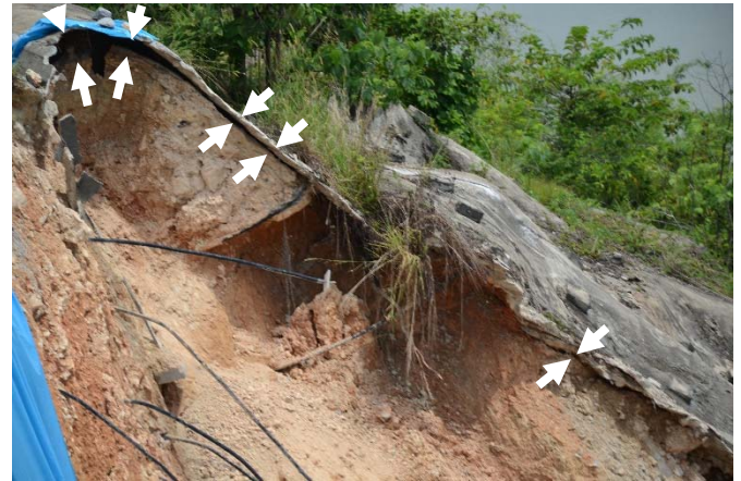
Figure 21 Gap Formation between Soil Nailed Slope and Shotcrete Facing
