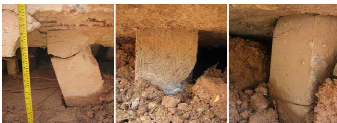
Figure 18 Settlement of piling platform and flexural damage of embankment foundation piles
