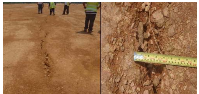
Figure 4 Longitudinal Crack found on the Embankment
