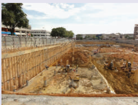
Figure (Top) – Initial stage of excavated platform - Residential Package
