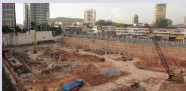
Figure (Top) - Initial stage of excavated platform - Retail Package
