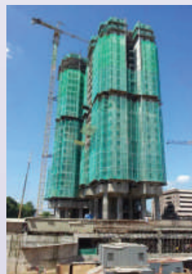
Figure (Top) - Construction of superstructure - Residential Package (Architect: DES Architect)
