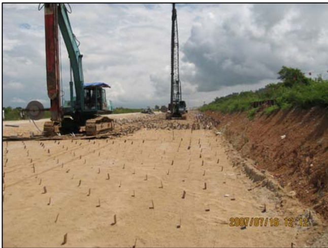
Typical PVD Machine working beside the Live Track
