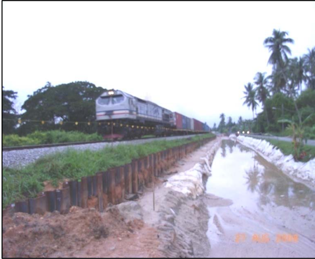
Typical Cross Section and Photo showing Temporary Sheet Pile for E&R.
