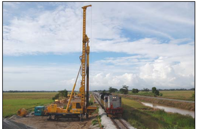
Installation of Stone Columns adjacent to Existing Live Track.
