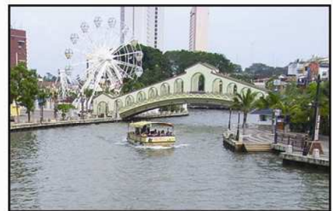
Figure 11: Old Bus Station Pedestrian Bridge Completed in January 2010
