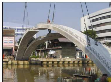
Figure 2 : Launching of Bebo Arch Frame
