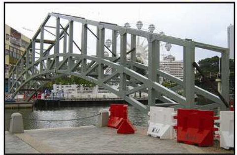
Figure 10: Steel Arch Frame Upon Launching
