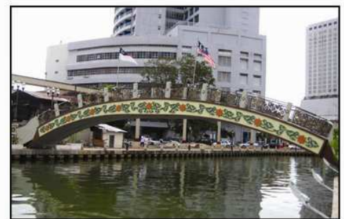
Figure 3: Kampung Mortern Pedestrian Bridge Completed in December 2009
