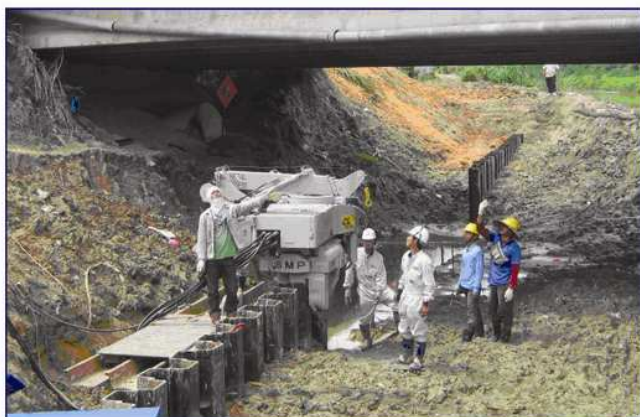
Figure 4: Use of "press-in" sheet piling method
