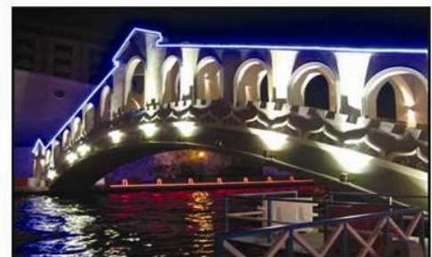
Figure 12: Night view of Old Bus Pedestrian Bridge
