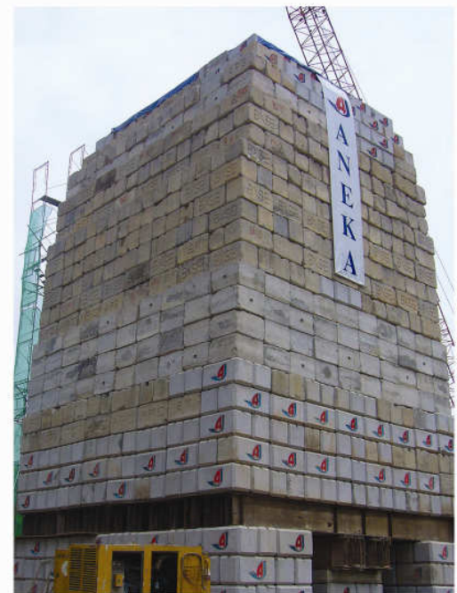
Instrumented Test Pile C
