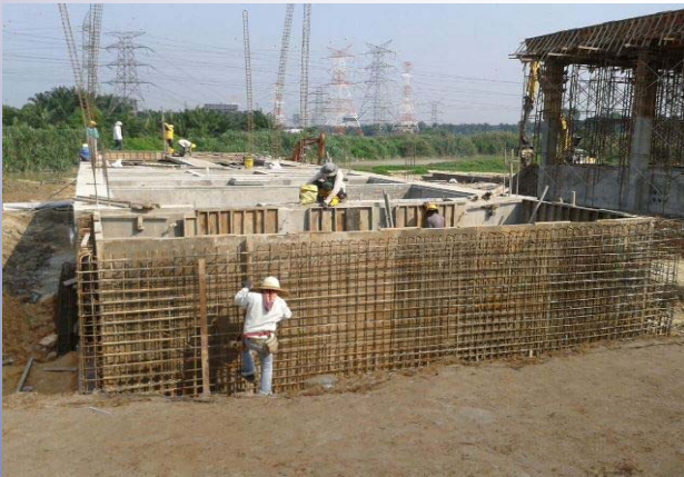
Figure (Top) – Mid Stage Concreting for Pumping Station
