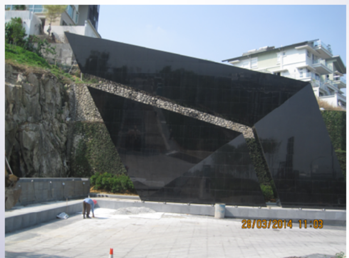
2014.03.28 : OVERALL WORK COMPLETION
