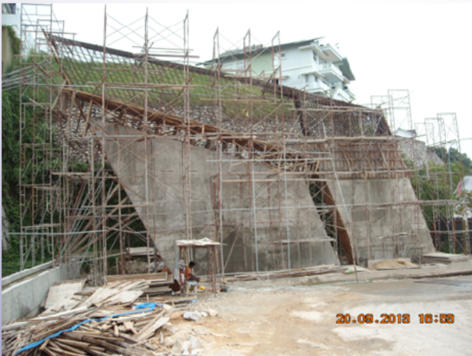
2013.09.20 : STAGE CONCRETING
