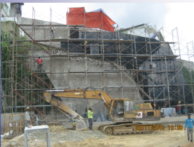
2013.11.22 : GRANITE FINISHES INSTALLATION
