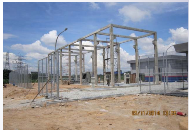
Figure (Top) – Completion of Sg. Langat Pumping Station
