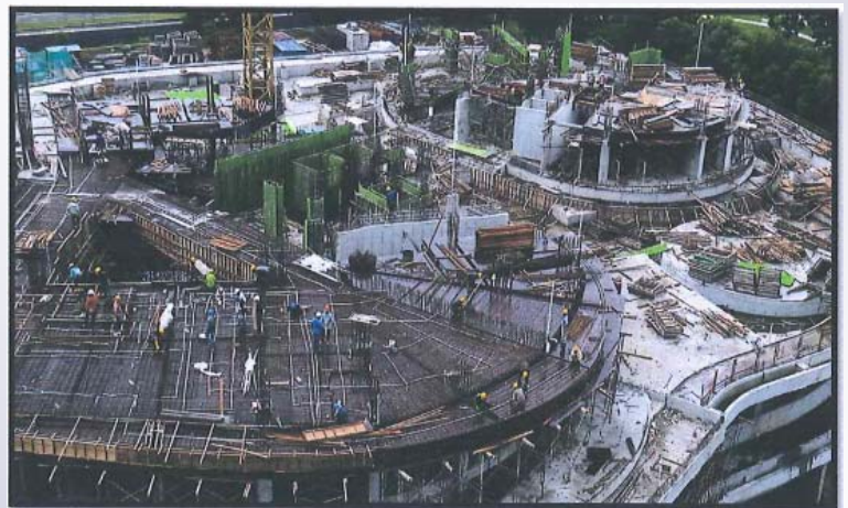
Figure 3: Block D1 & D2 Podium Floor Complete Cast and Condominium Floor Circular Beam construction W.I.P.
