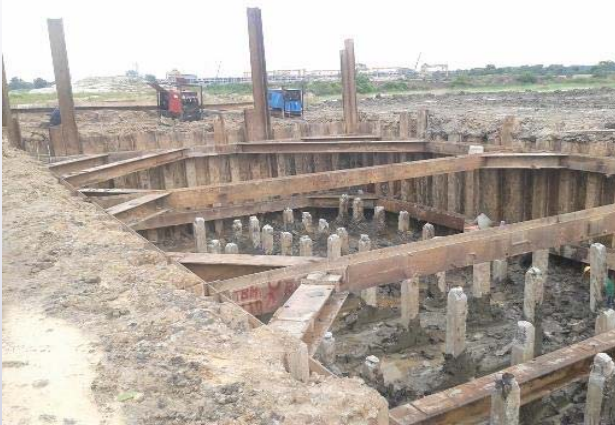
Figure (Top) – Cofferdam deep excavation for Pumping Station
