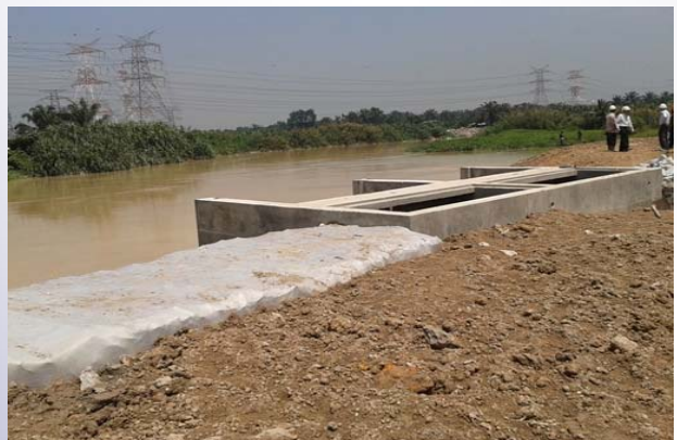
Figure (Top) – Final Stage of Intake Structure
