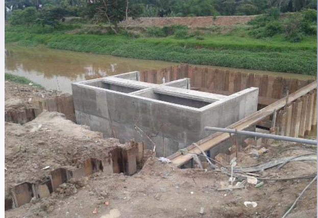
Figure (Top) – Cofferdam for Intake Structure
