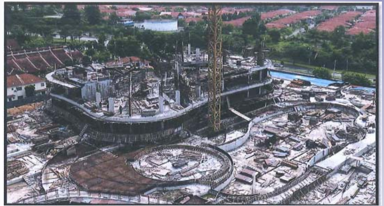
Figure 2: Block C and Podium Swimming Pool under construction
