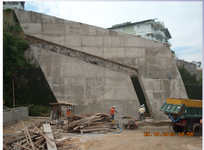
2013.10.25 : R.C. WORKS COMPLETION
