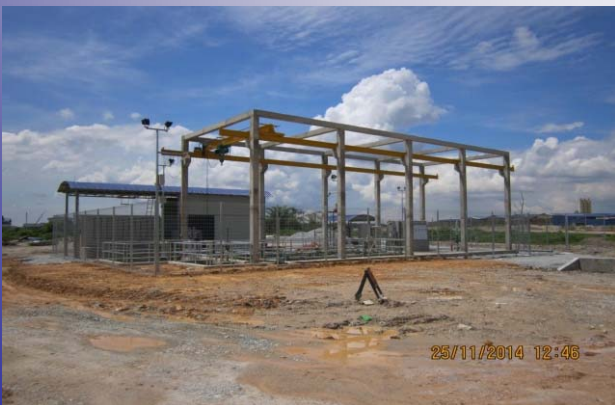
Figure (Top) – Completion of Sg. Labu Pumping Station
