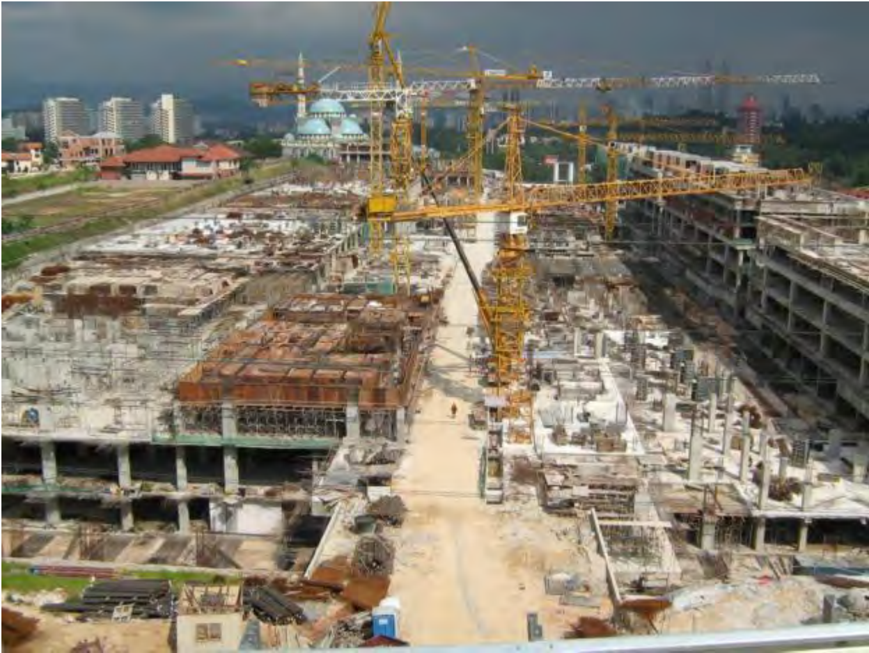
Figure 11: Picture taken after completion of basement construction.
