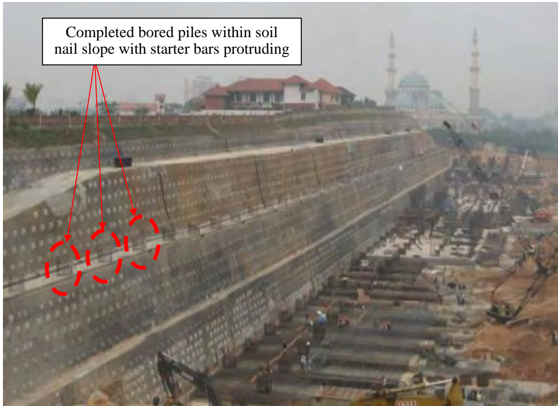
Figure 9: Picture taken after completion of soil nailing works and basement construction on-going.
