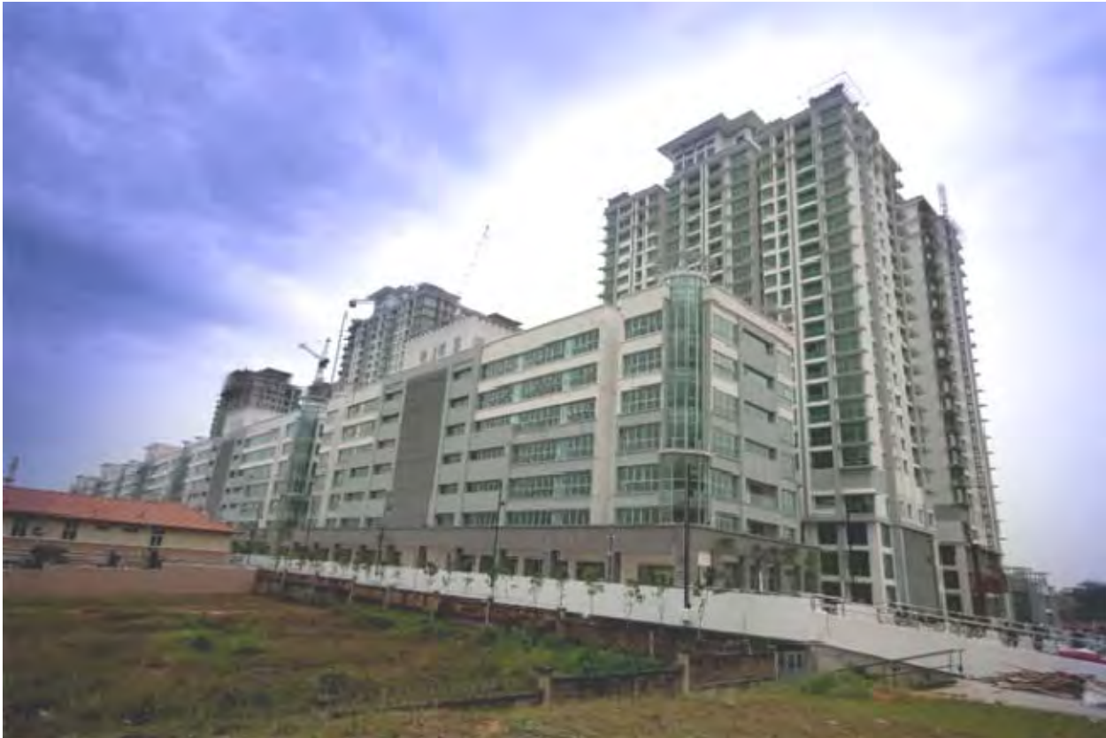
Figure 3: Completed basement and superstructure works.
