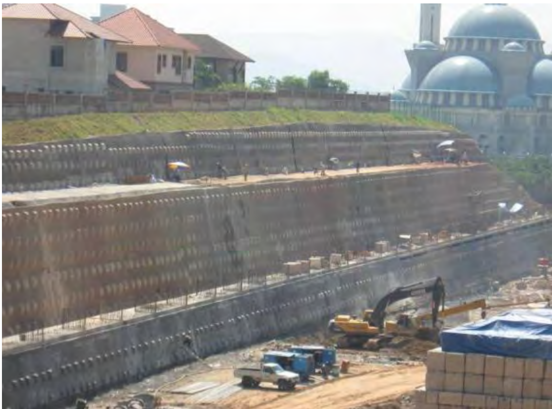
Figure 9: Picture taken after completion of soil nailing works and basement construction on-going.
