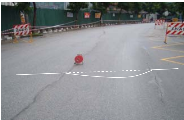
Fig. 15. Subsidence trough developed on the retained ground.
