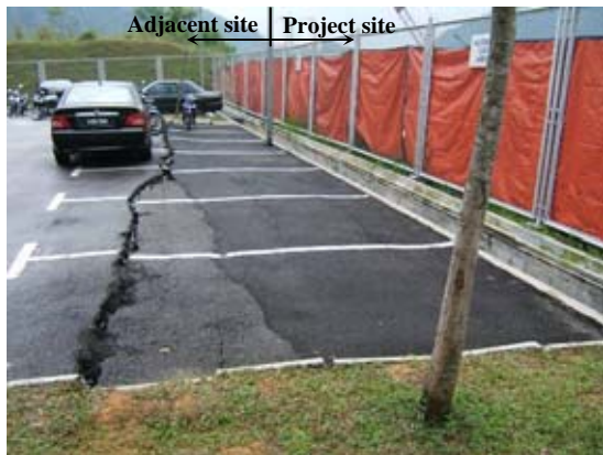
Fig. 22. Site conditions of adjacent lot after the incidence of wall and ground distresses (Northern view).
