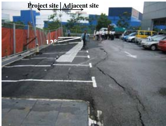
Fig. 21. Site conditions of adjacent lot after the incidence of wall and ground distresses (Southern view).
