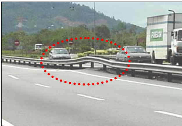
Fig. 13. Hump over Piled Culvert (After Gue, 2000)
