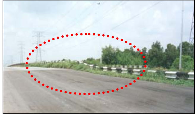
Fig. 9. Hump at Bridge Approach (After Gue, 2000)
