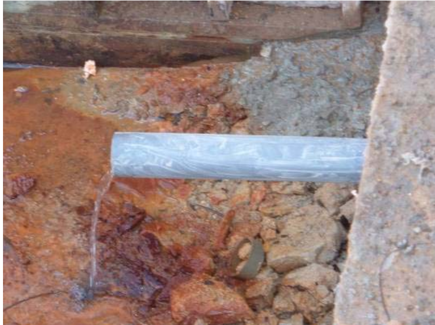
Fig. 24. Continuous seepage flow collected in Subsoil Drains.
