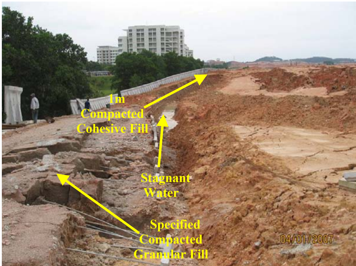
Fig. 48. Collapsed Reinforced Soil Wall
