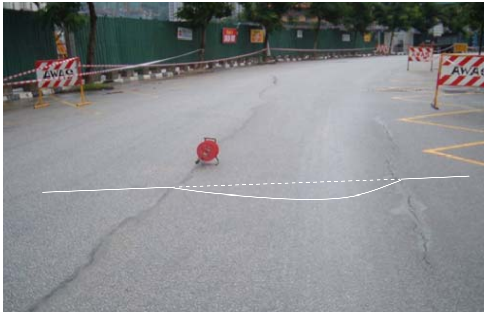
Fig. 30. Subsidence trough developed on the retained ground.
