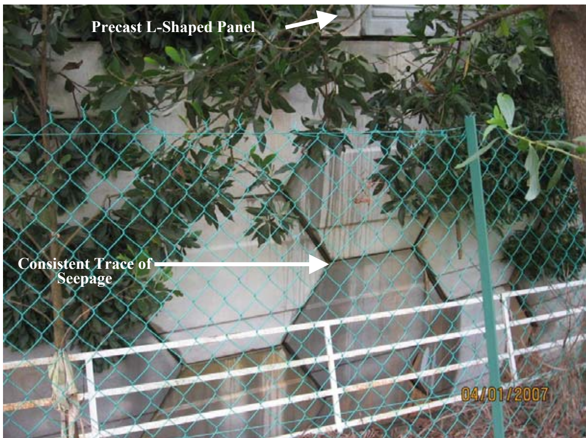
Fig. 49. Sign of Water Seepage on Top Wall Panels
