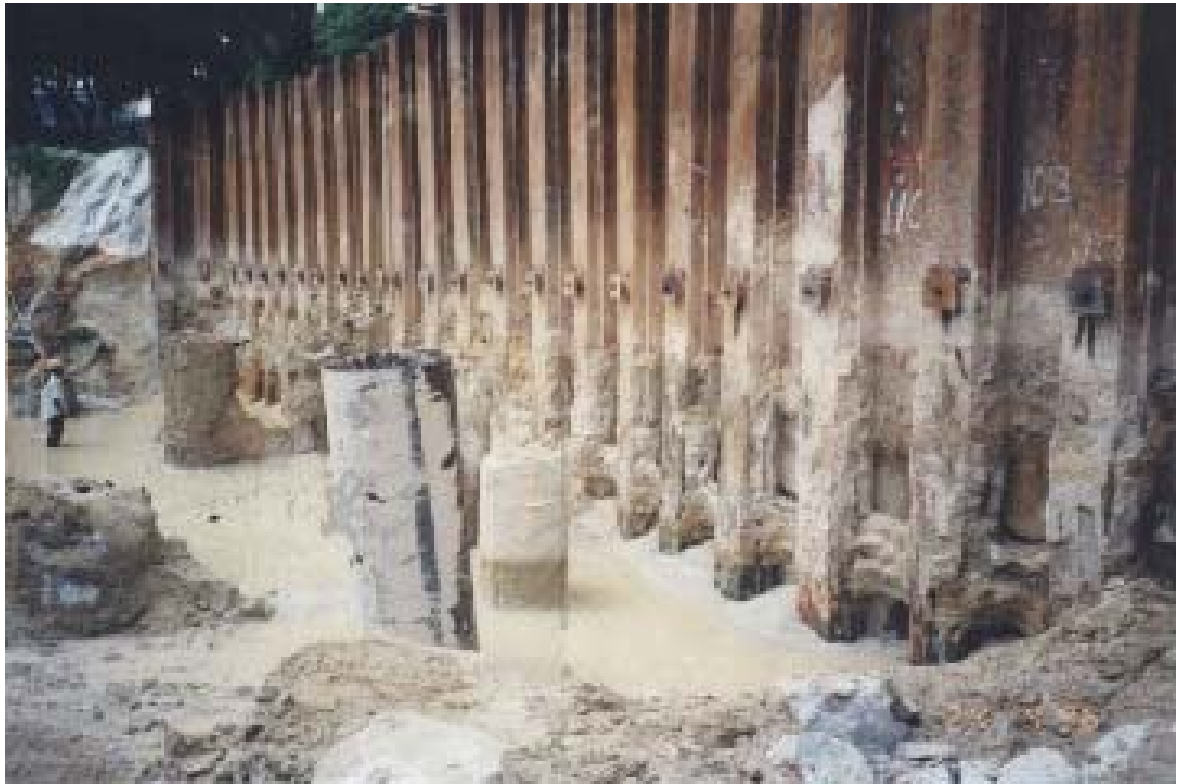
Fig. 4. View of Retaining Wall with Jacked-in pipe Anchorage.
