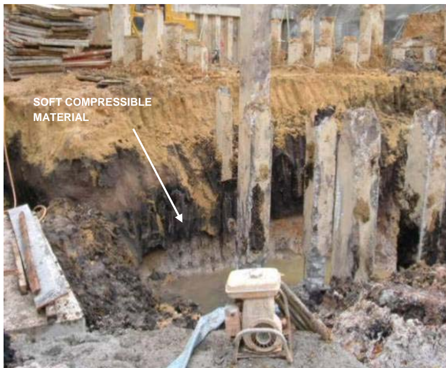
Fig. 25. Soft compressible material detected at localized pile cap excavation.
