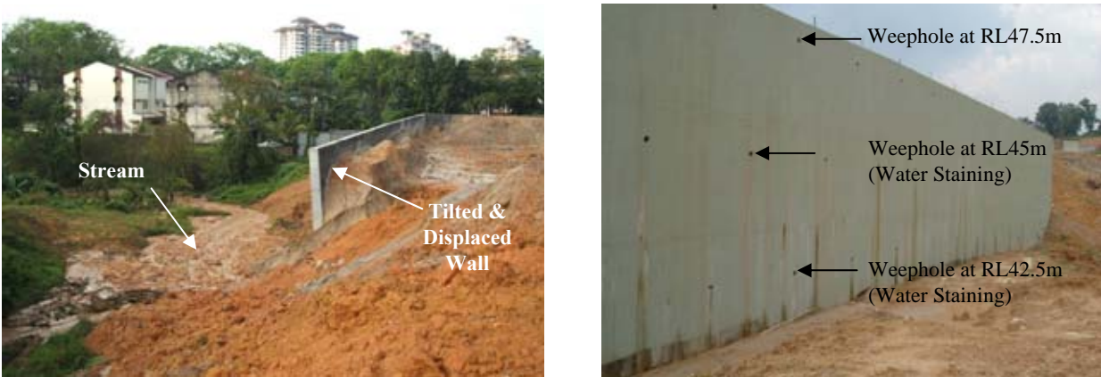
Fig. 45. Overall Site Conditions and Water Staining at Weephole Drains
