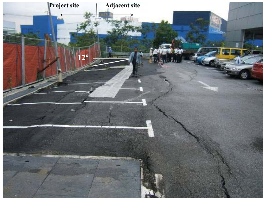
Fig. 36. Site conditions of adjacent lot after the incidence of wall and ground distresses (Southern view).
