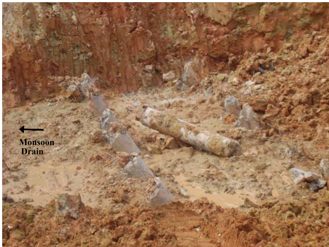
Fig. 50. Pile Head Connection Exposed after Removal of Collapsed Debris
