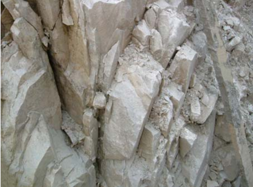
Figure 7: Vertical joints in exposed limestone in the Kuala Lumpur area.
