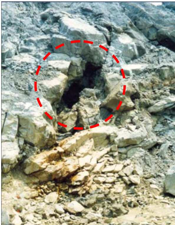
Figure 5: Cavern/cavity exposed after excavation.
