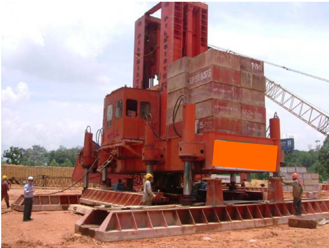
Figure 8: A typical hydraulic jacked-in piling system used in Malaysia.
