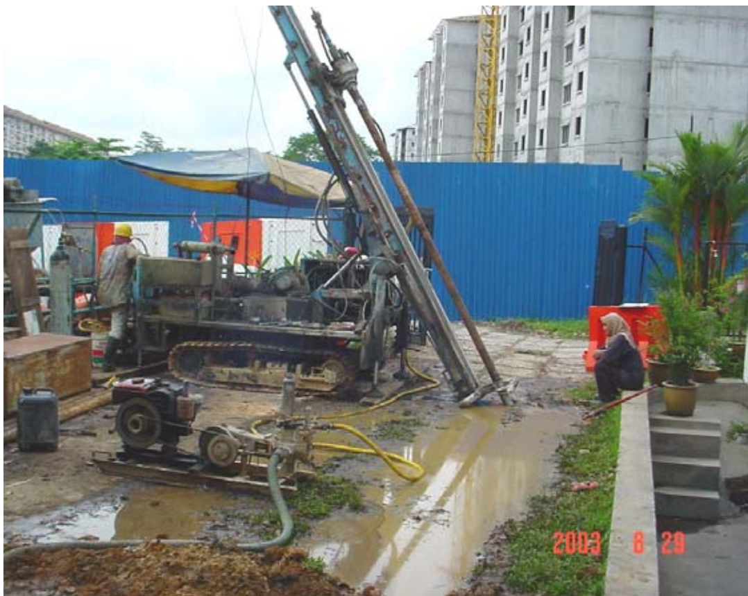
Figure 17: Typical drilling machine and pump for cavity treatment using grout/mortar.
