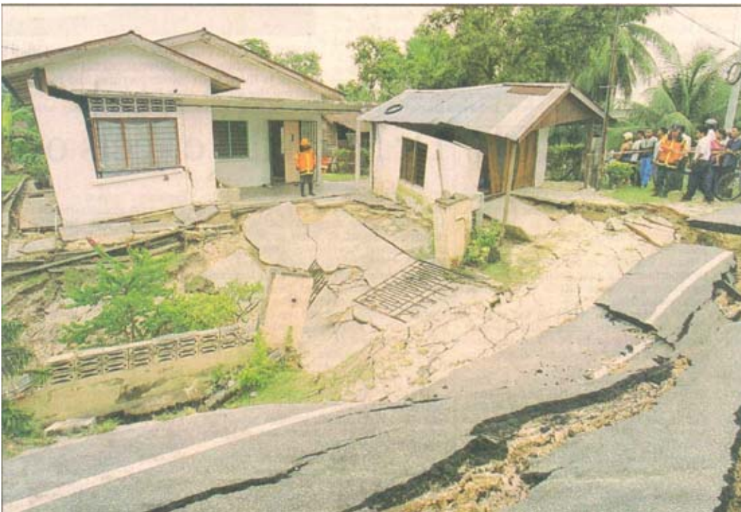
Figure 3: Sinkhole near Ipoh, Perak.
