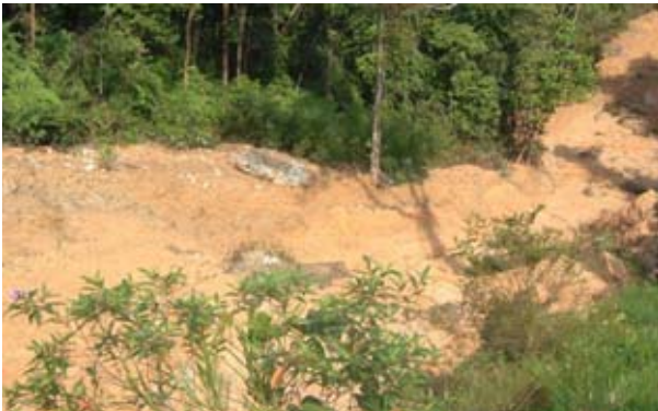
Fig. 13. Travel of Debris and Failed Mass Downhill
