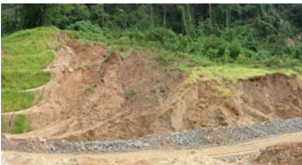
Fig. 8. Front View of Failed Slope
