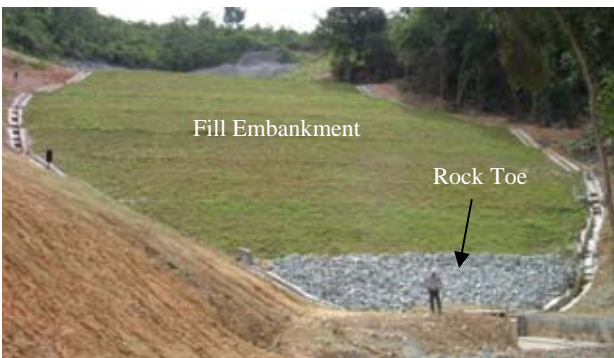
Fig. 14. Completed View of Filled Embankment
