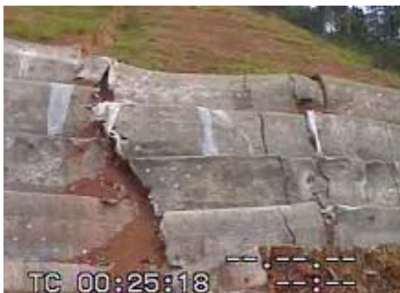
Fig. 4. Front View of Failed Slope
