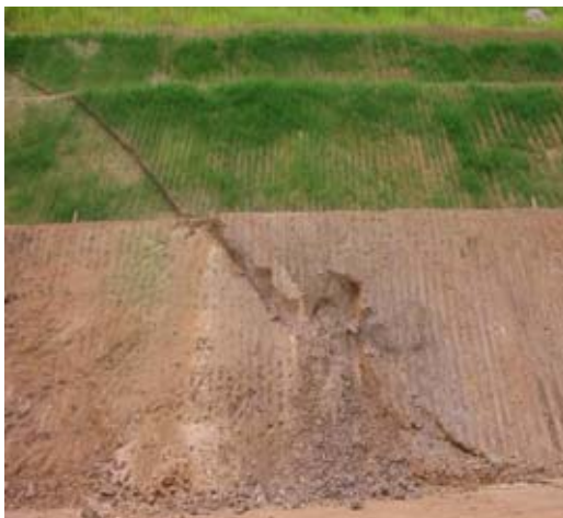
Fig. 11. Localised Failure of Slope
