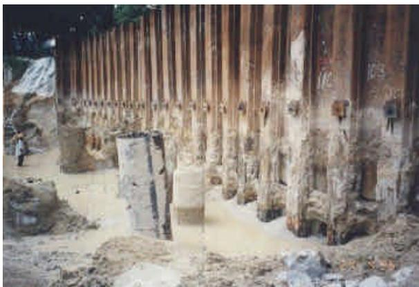
Figure 2 : The Installed Jack-In-Pipe Anchorages at the Sheet Pile Retaining Wall of 9m High
