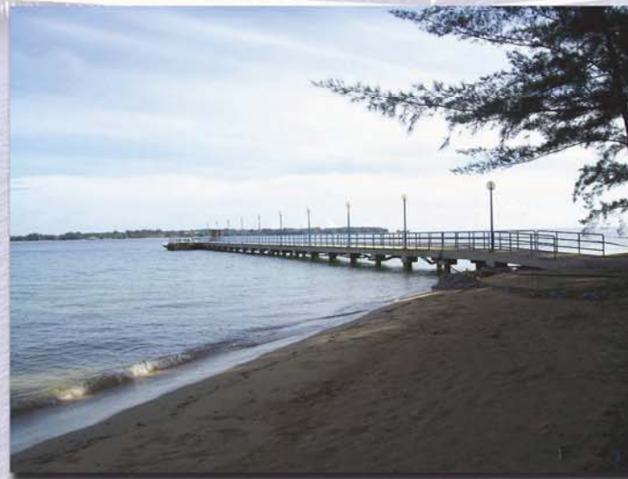
For jetty, there are "T", "I" and "L" shape arrangement for berth. It could also be floating, on pile or wharf arrangement.
