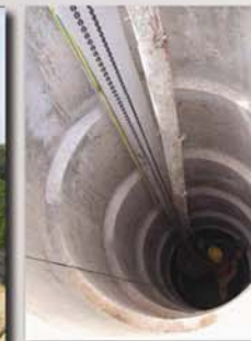
Concrete linings to support dug hole
