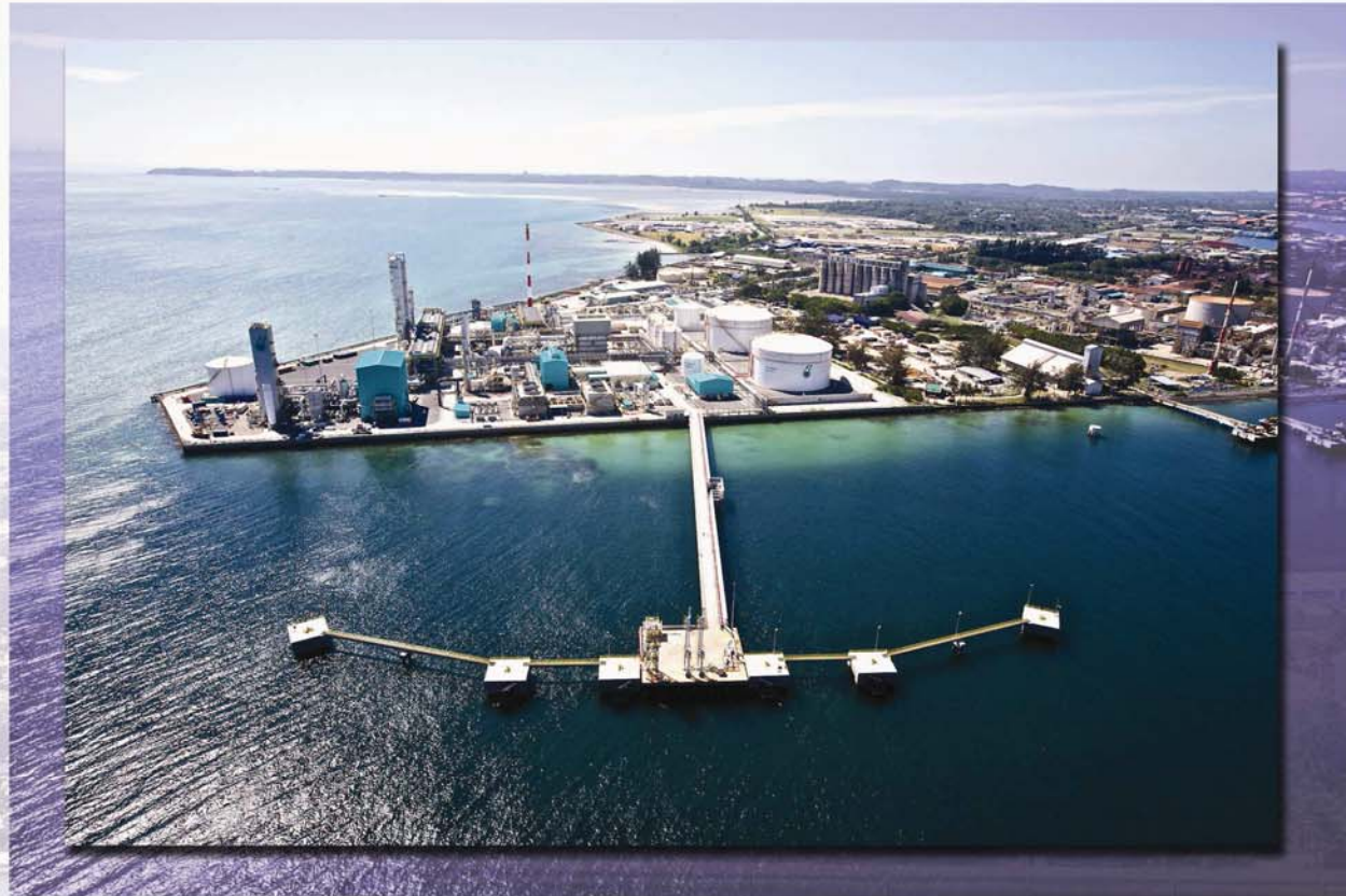
7 Islands berth are required to cater for Chemical Tanker mooring for approximately 1-2 days.
