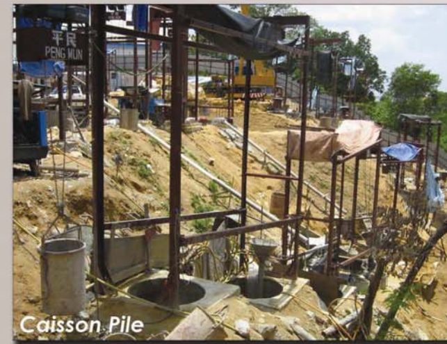
Concrete linings to support dug hole
