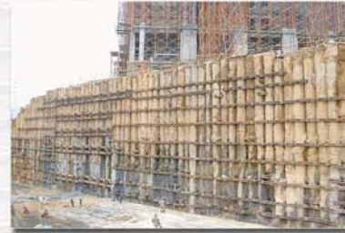
Cut & Cover LRT Tunnel, Putra Jaya
