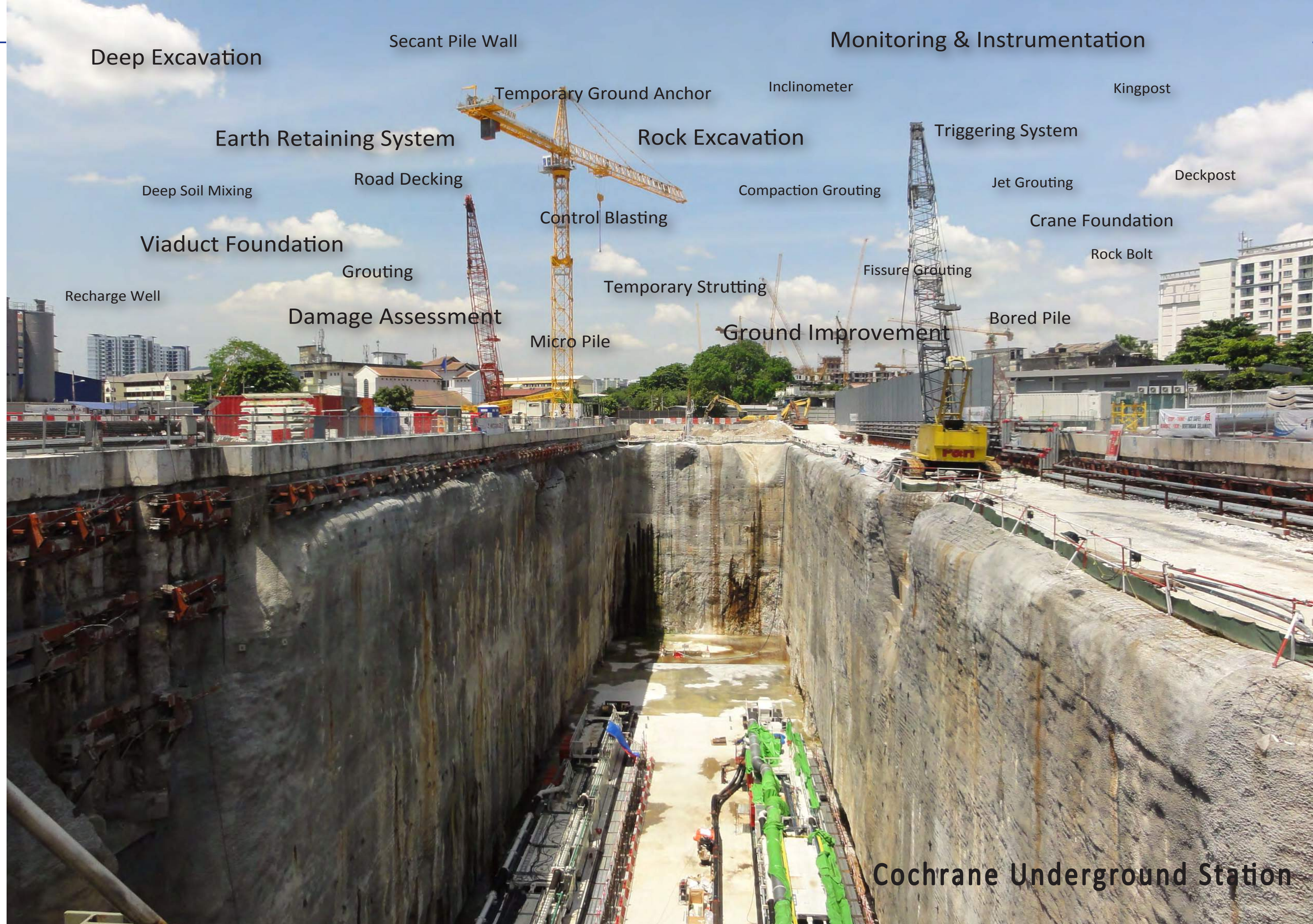
Temporary Ground Anchor as temporary support of secant pile wall
