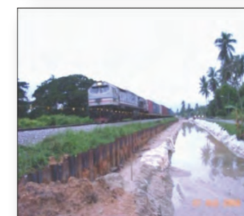
Top: Temporary Sheet Pile for Excavation and Replace Method (E&R).
