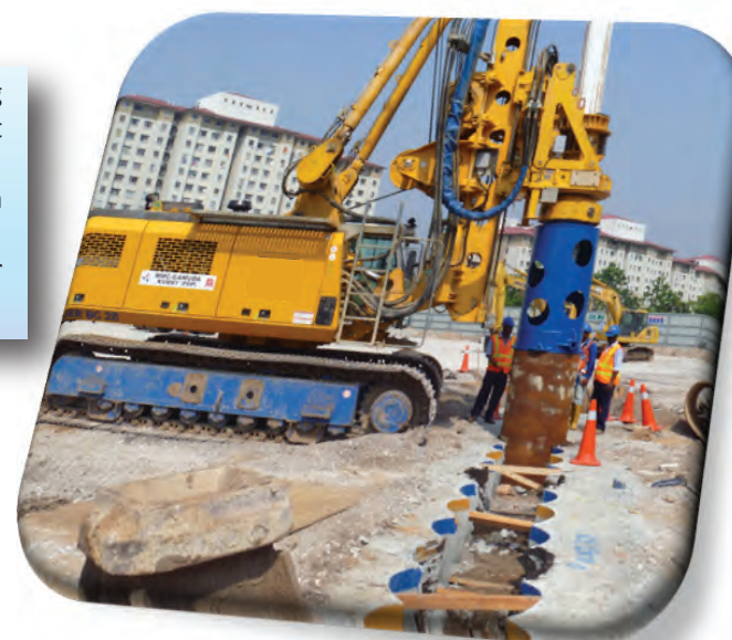
Installation of Secant Pile Wall
