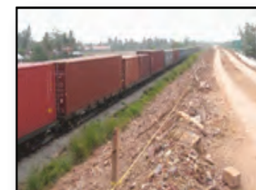
Right: Embankment fill with surcharge next to existing live tracks
