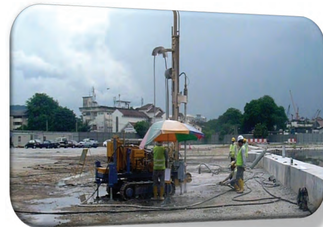
Rock Fissure Grouting
