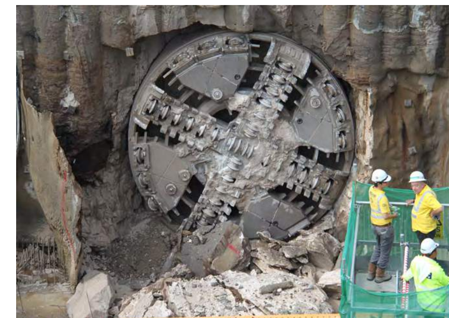
Variable Density (VD) TBM Breakthrough at Maluri South Portal
