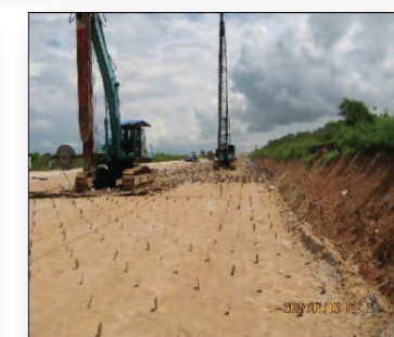
Top: Typical PVD Machine working beside the Live Track
